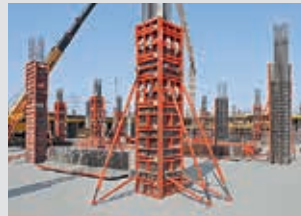
Column Formwork
