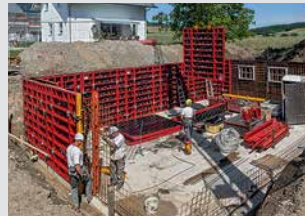
Wall Formwork
