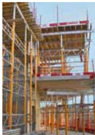
An arrangement of MULTIPROP Strike-and-erect falsework utilising aluminium beams as primary girders.
