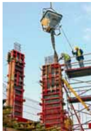
Pouring of one of the TRIO columns.
