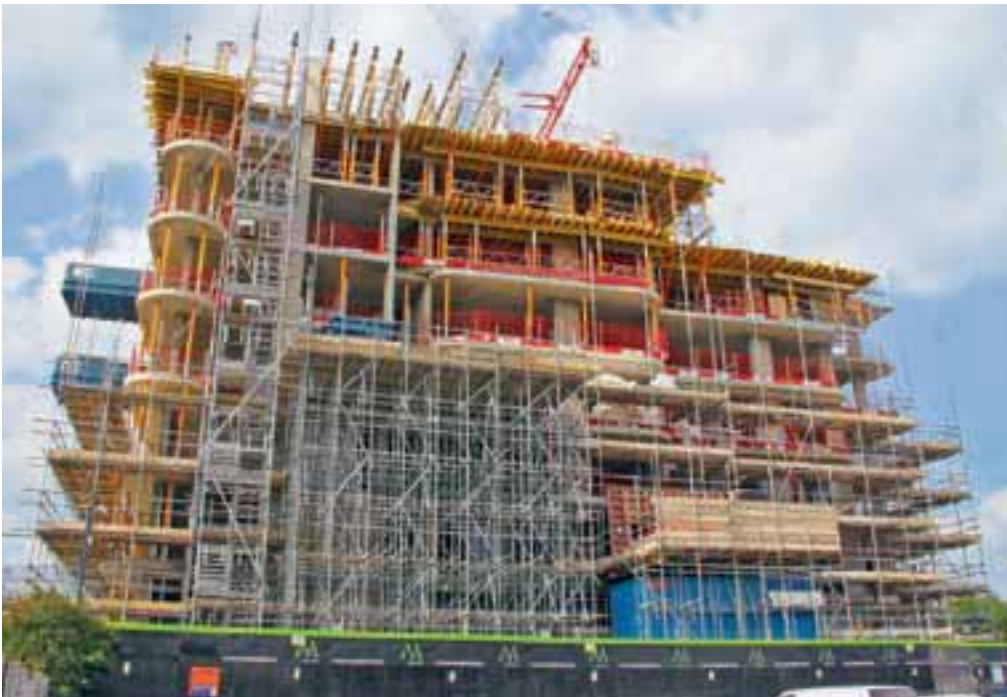
TRIO panel wall formwork used to form the columns. Formwork erection and pouring of ten columns could be carried out in one day by a two man team.
