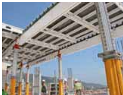
SKYDECK panel slab formwork.
