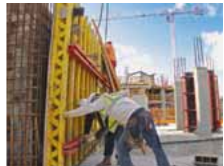
Positioning of the VARIO panels by site personnel.
