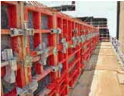
Clear safe access provided by FB 180 working platforms.
