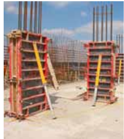
TRIO panel wall formwork used to form the columns. Formwork erection and pouring of ten columns could be carried out in one day by a two man team.
